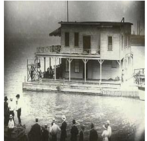
ABOVE: Just like today, the SYC clubhouse underwent many changes. Here we see the Clubhouse, approximately 1920, minus the rooftop dance floor as well as an open second floor veranda.
