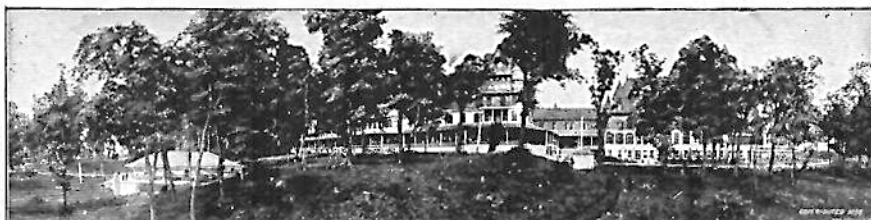
View of the old Victory Hotel
