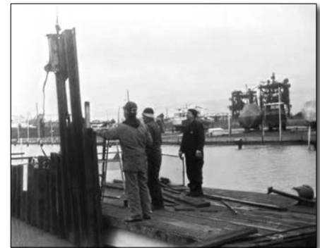
Docks and seawalls were built with the help of members.
